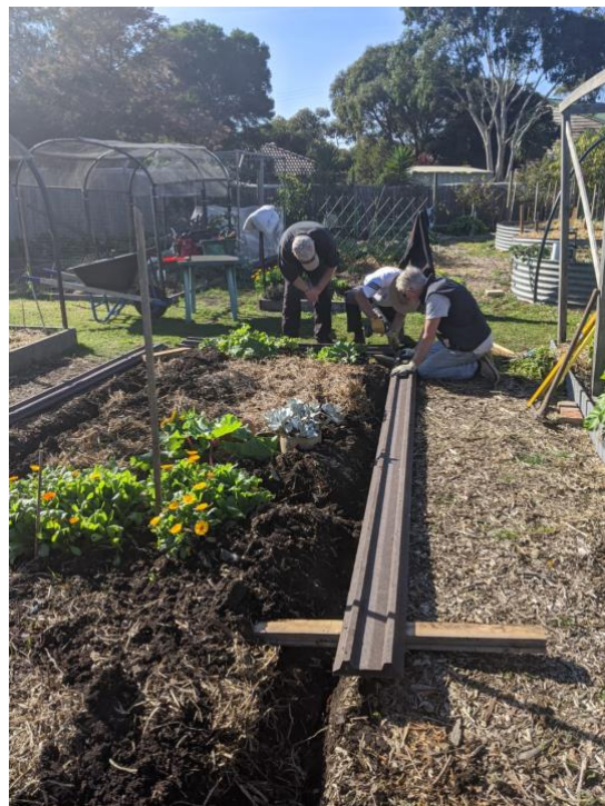
The construction team – John, Bruno and Michael installing the recycled garden plot edging boards.
