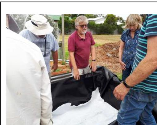
After the plastic add another layer of geotech to protect plastic from the scoria. Now the inlet water pipes are installed.
